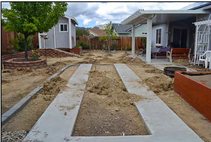
Our Backyard Renovation in Process
